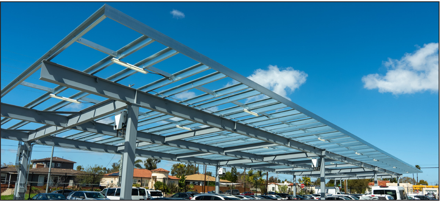
Progress after phase one — the completed canopy over the faculty lot that will house solar panels. Jameson Grohman ('26)
