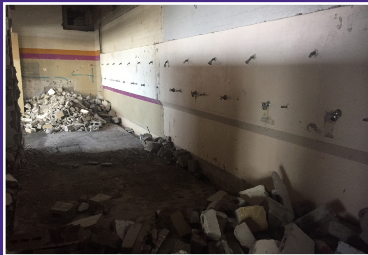
By mid-August here’s what was left of the old gym showers.
