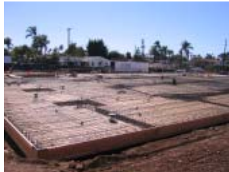
Ready to Pour the Foundation/Deck November 6, 2006
