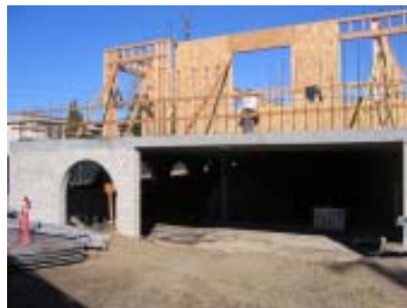
Entrance to Parking Structure and 1st Wall of Western Building January 1, 2007
