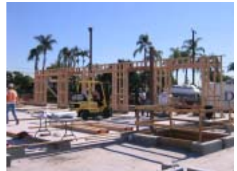
The framing of the first wall is erected. December 1, 2006
