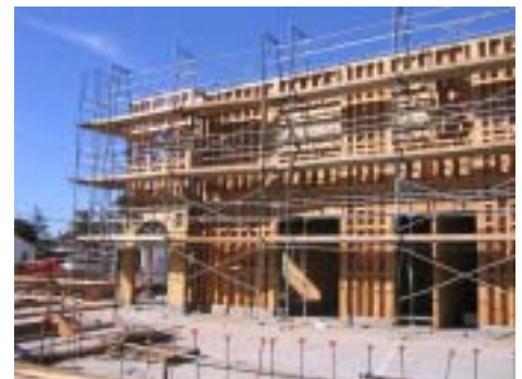
Framing of Eastern Building January 23, 2007
